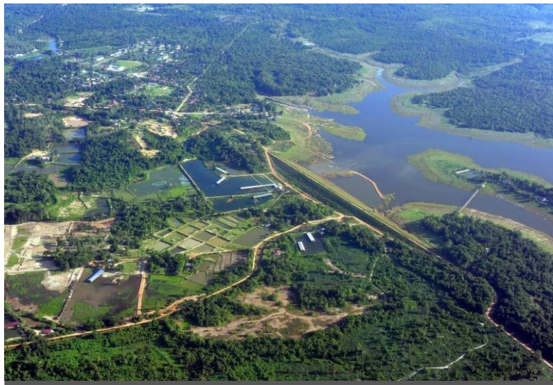
Nam Houm Irrigation Reservoir
